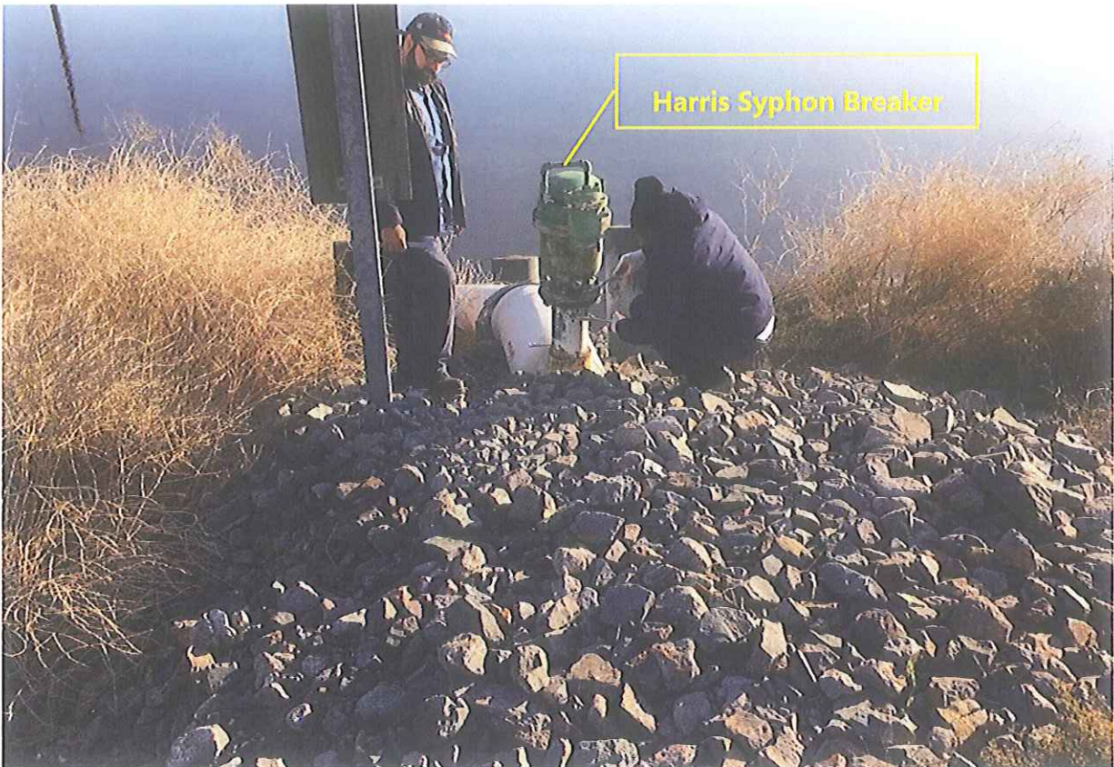
Photo A Old River West Bank (looking NW)
