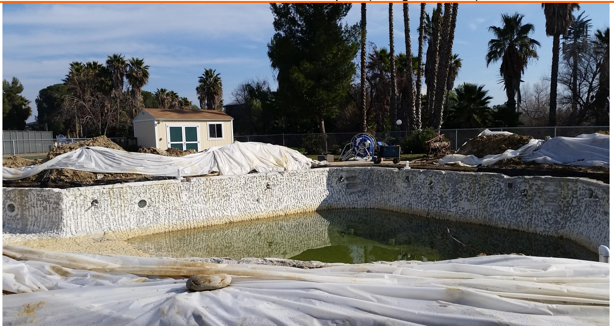
Photo 4 – West side of the pool (facing east)
