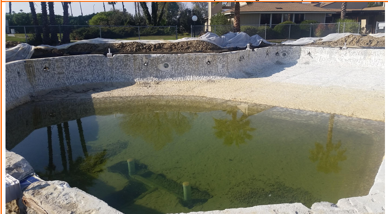
Photo 2 – Southeast side of the pool (facing west)
