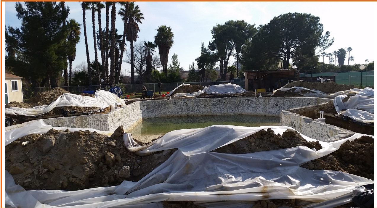
Photo 1 – Northwest side of the pool (facing southeast)
