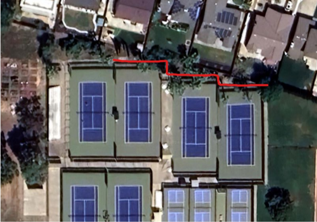
Area in Red Showing Approximate Location of Failed Retaining Wall
