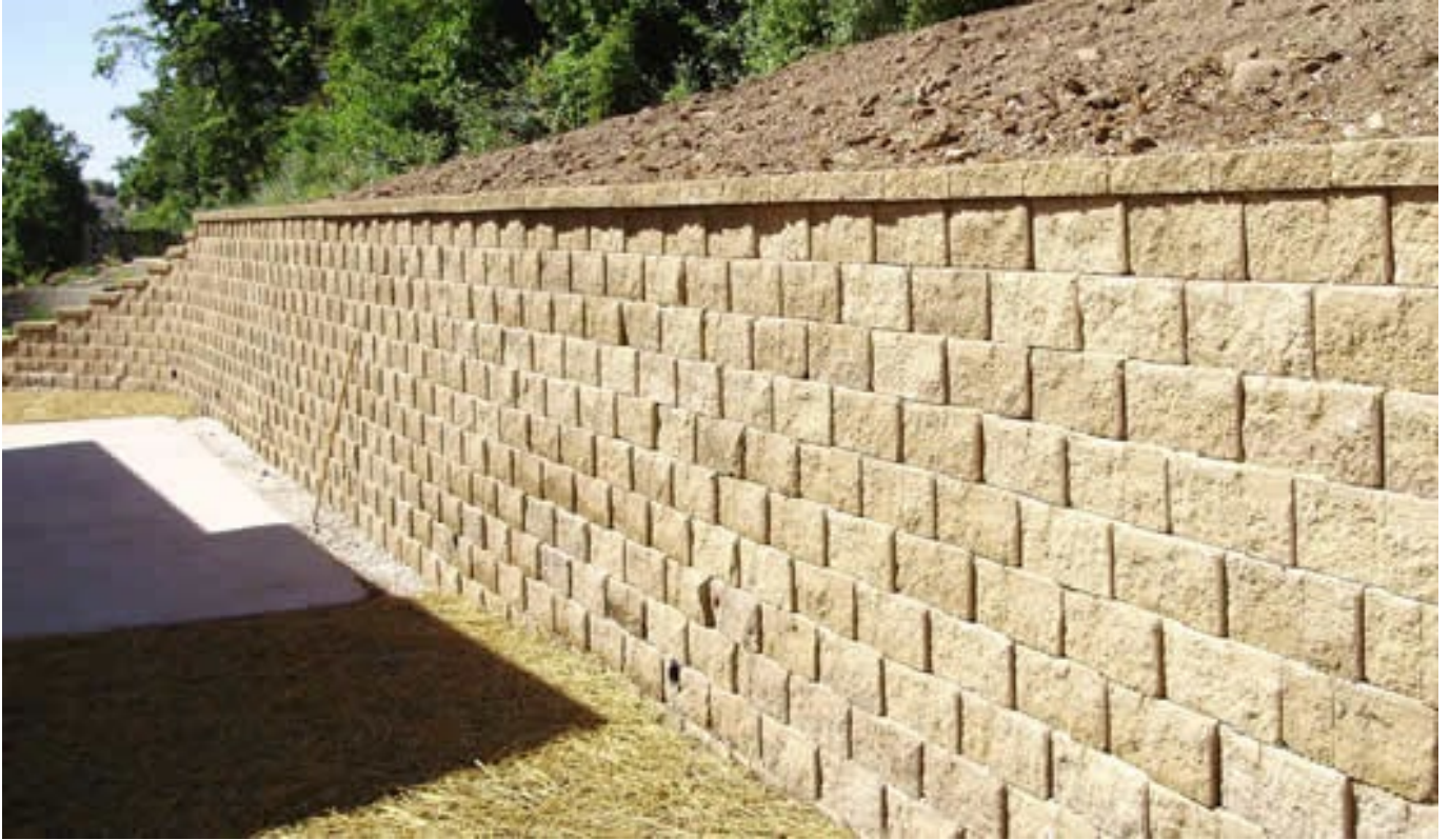
Example Keystone Style Stacked Block Retaining Wall
