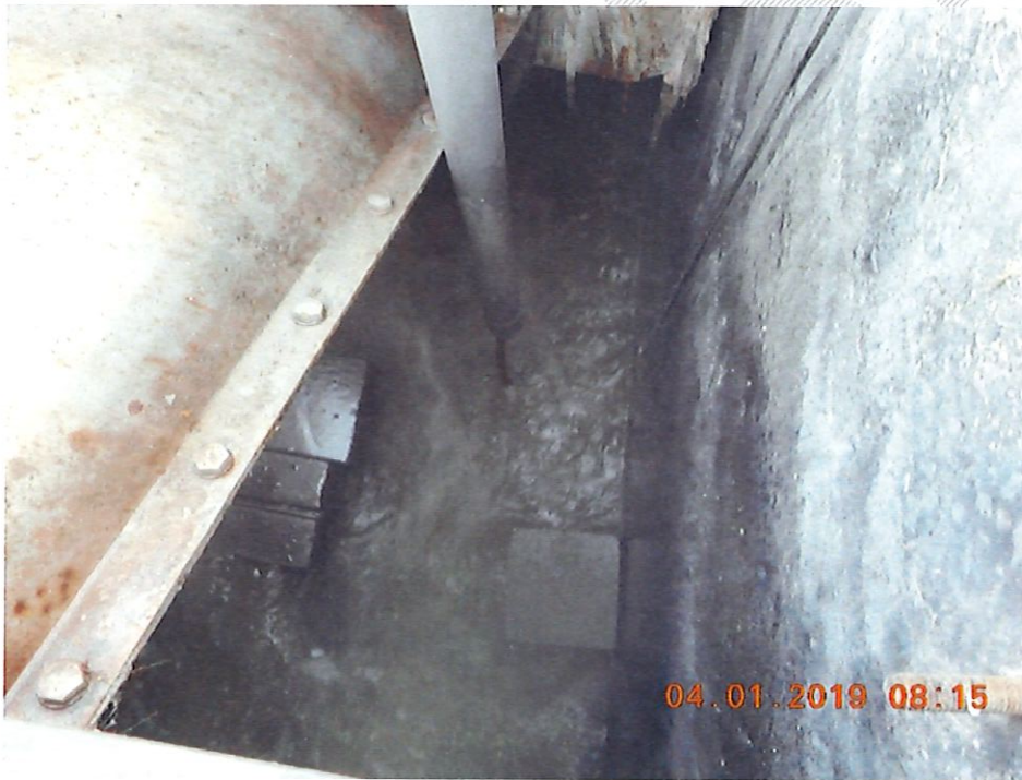
Figure 5-13 Initial Configuration of Concrete Blocks and Sampler Intake Tube in Screen Channel on 4-1-2019
