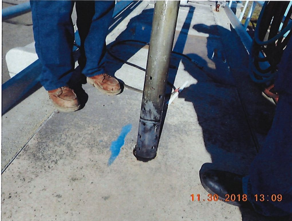
Figure 5-9 Perforated Pipe Surrounding Sampler Intake Strainer
