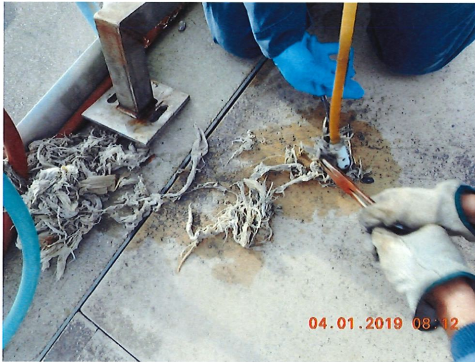
Figure 5-12 Rags Being Removed from Portable Sampler Intake Strainer on 4-1-2019
