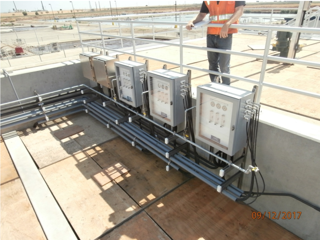
Figure 2 - EcoWash ACP NEMA 4X Air Control Panels, 3 Per Side, Total of 6.
